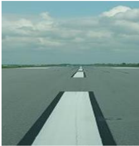
Figure A3.12. (NFARS) NFARS Taxiway Centerline Marking.
