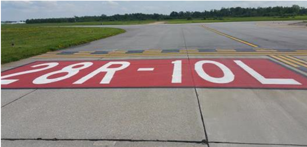
Figure A3.10. (NFARS) NFARS Taxiway/Taxiway (Intersection) Holding Position.
