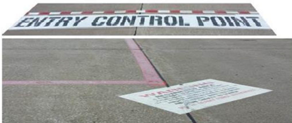
Figure A3.13. (Added-NFARS) NFARS ECP and Restricted Area Markings.
