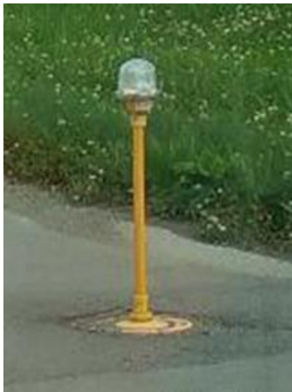
Figure A3.7. (NFARS) NFARS Runway Edge Light (yellow color last 2,000 feet).
