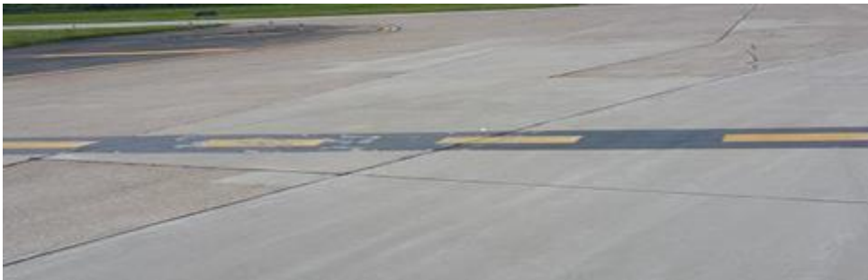
Figure A3.10. (NFARS) NFARS Taxiway/Taxiway (Intersection) Holding Position.
