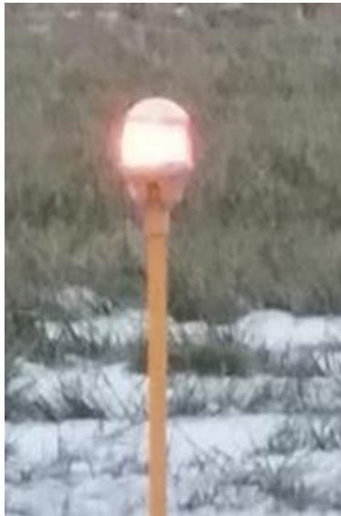
Figure A3.7. (NFARS) NFARS Runway Edge Light (yellow color last 2,000 feet).
