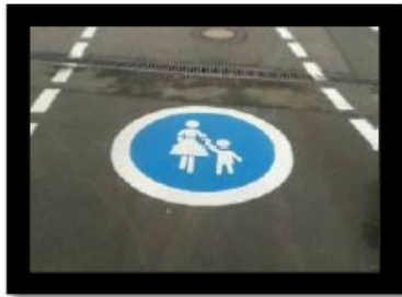
Figure 4.24. Pedestrian Cross Walks Denoted By Signs And/Or Markings.
