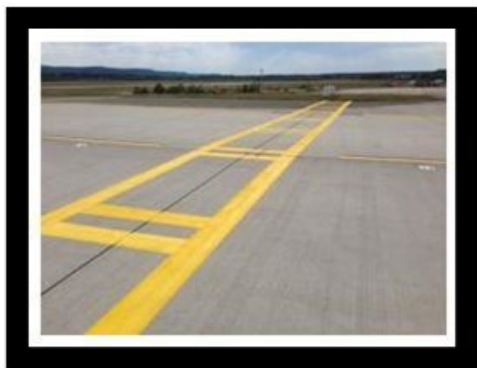
Figure 4.15. Instrument (INST) Hold Position Lines.
