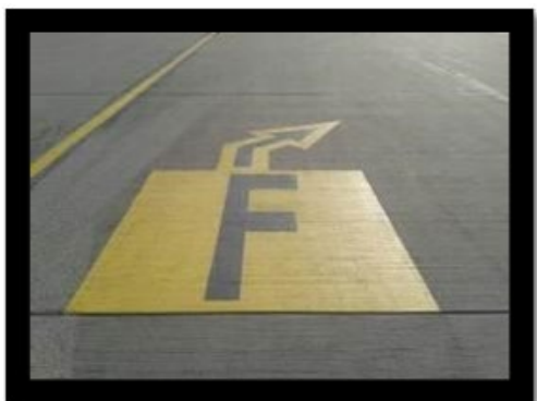
Figure 4.11. Surface Painted Direction/Location Signs.
