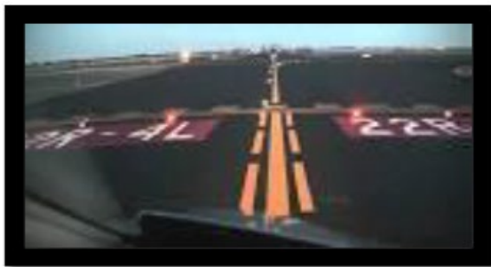
Figure 4.19. Stop Bar Lights.
