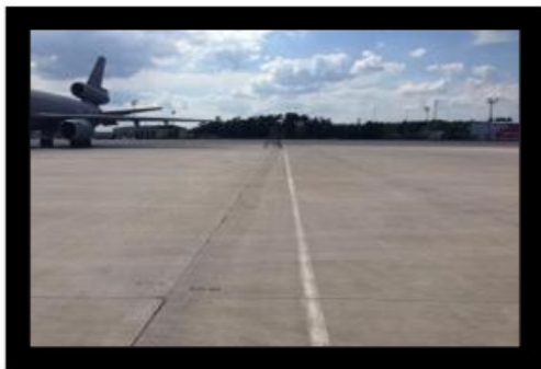
Figure 4.10. Wingtip Clearance Lines.
