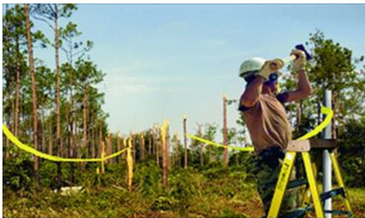
Figure 4.16. Setting Marker Poles and Tall Stakes.
