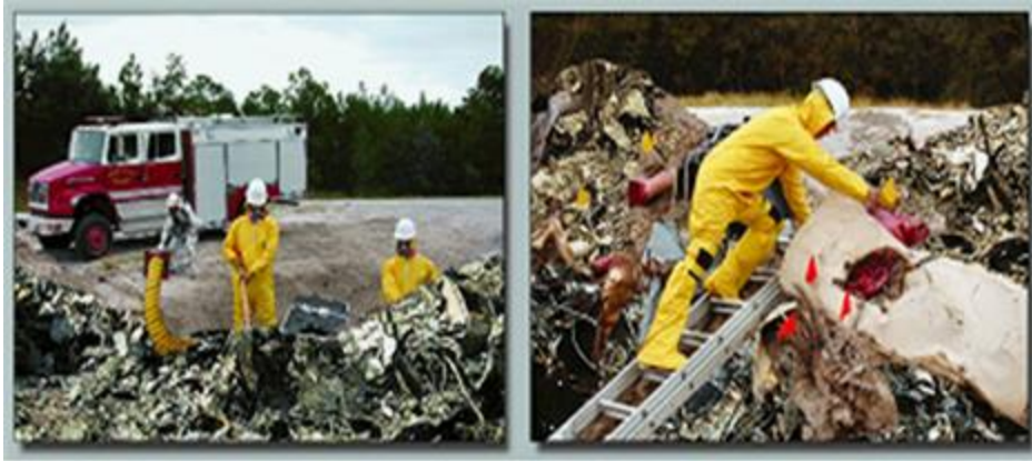
Figure 4.32. Take Precautions to Address Hazards in the Crater Such as Using Ladders, Ventilation, and Higher Levels of PPE.
